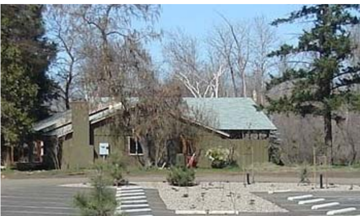
Newly completed Jefferson Nature Center, on the grounds of US Cellular Community Park in south Medford. Photo JNC Staff.
